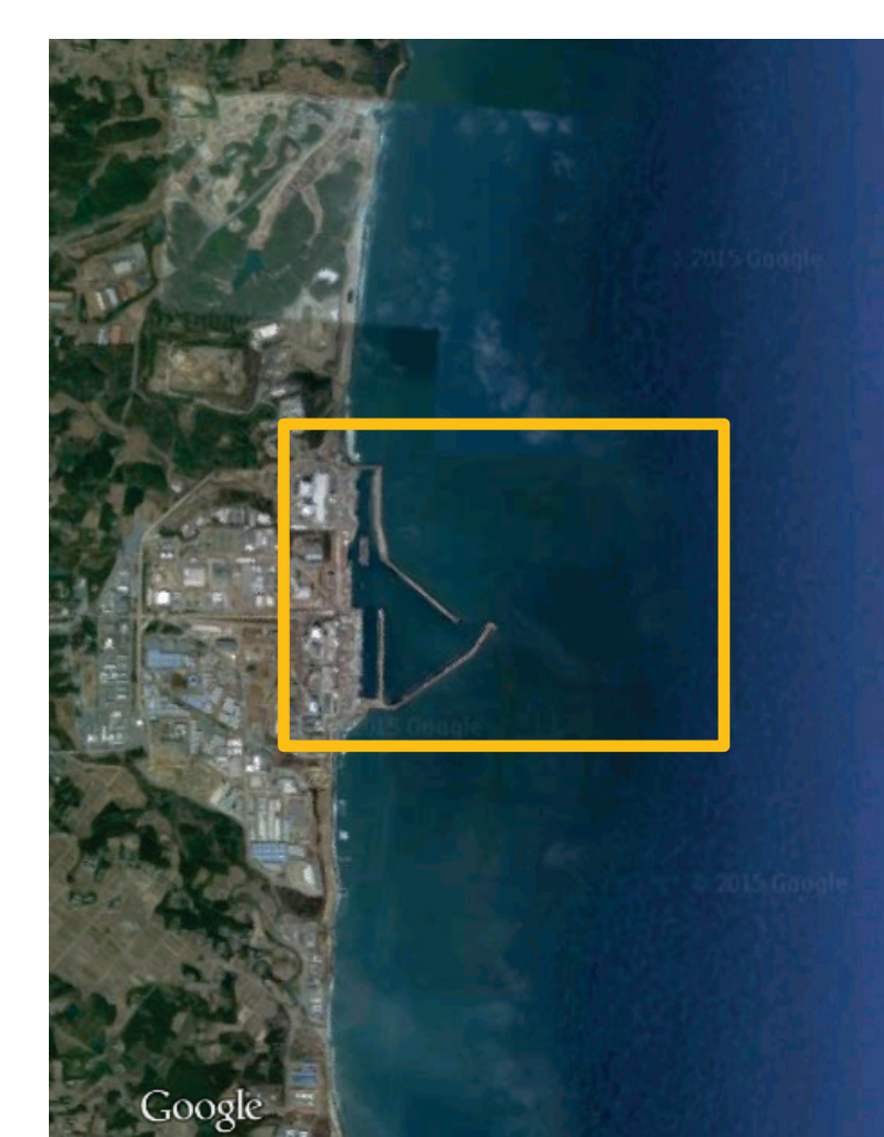
(a) Fukushima Daiichi Nuclear Power Station.
